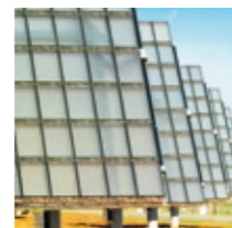
Concentrix Solar power plants at Puertollano and Seville (Spain), the first large power plants in Europe to use triple-junction solar cells.
