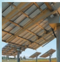
Concentrix Solar power plants at Puertollano and Seville (Spain), the first large power plants in Europe to use triple-junction solar cells.
